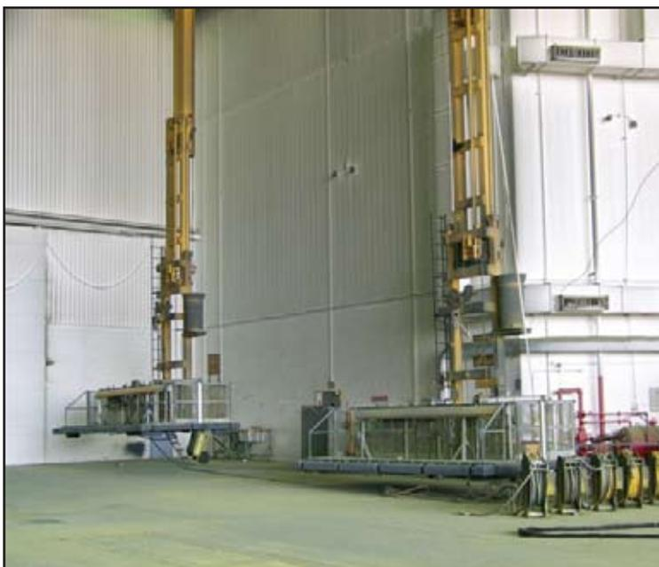
Paint booth crane in Tinker Air Force Base Hanger
